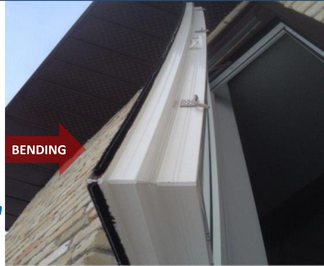
Time-limited performance of hollow frame structure (<20 years)
