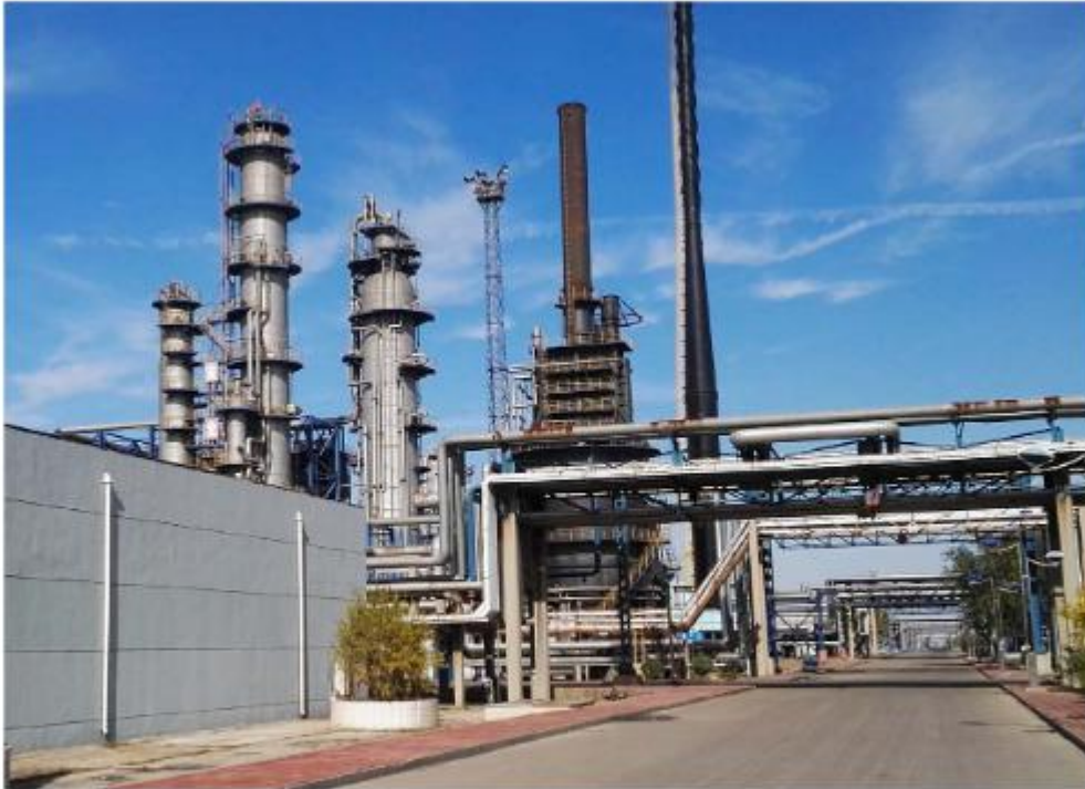
Industrial waste-gas management
