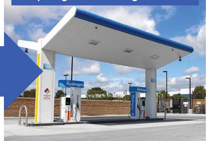
Hydrogen Refueling Station
