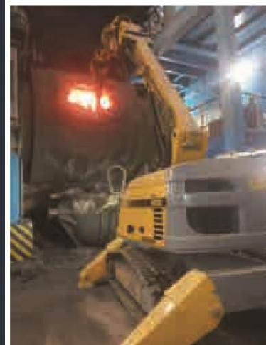
Brokk800清转炉口
